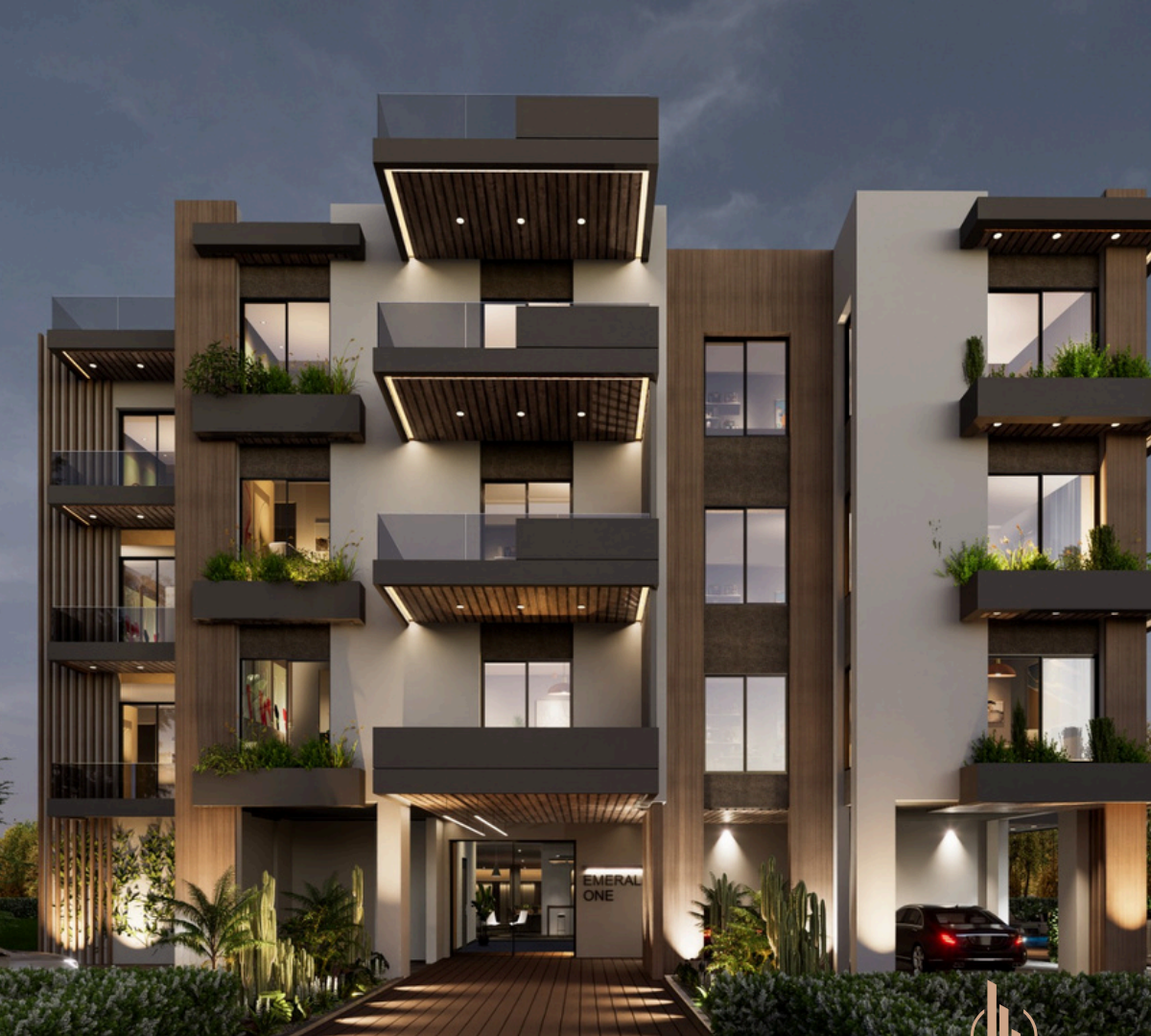
Facade Wide View
