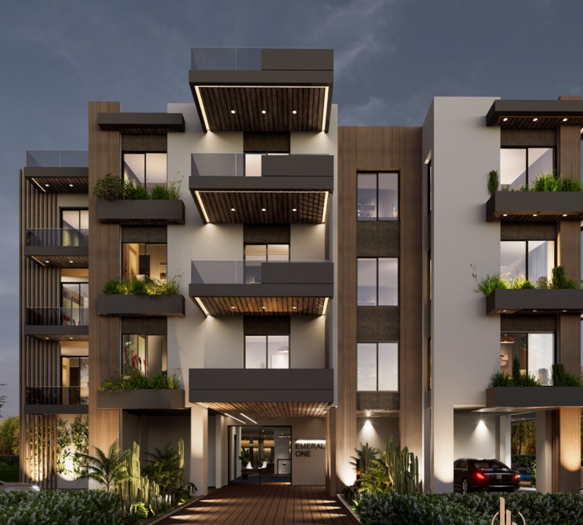
Facade Wide View
