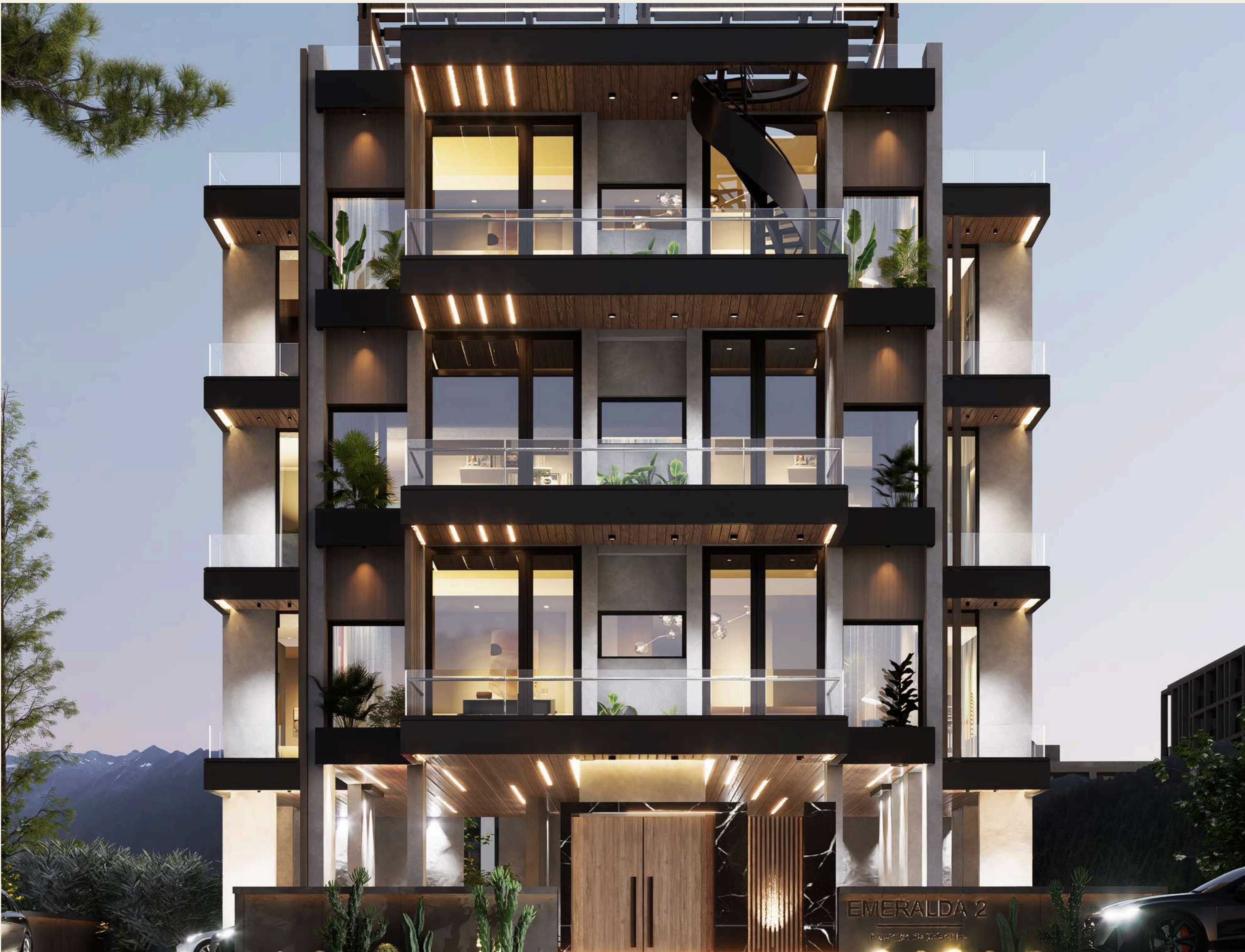
Facade Wide View
