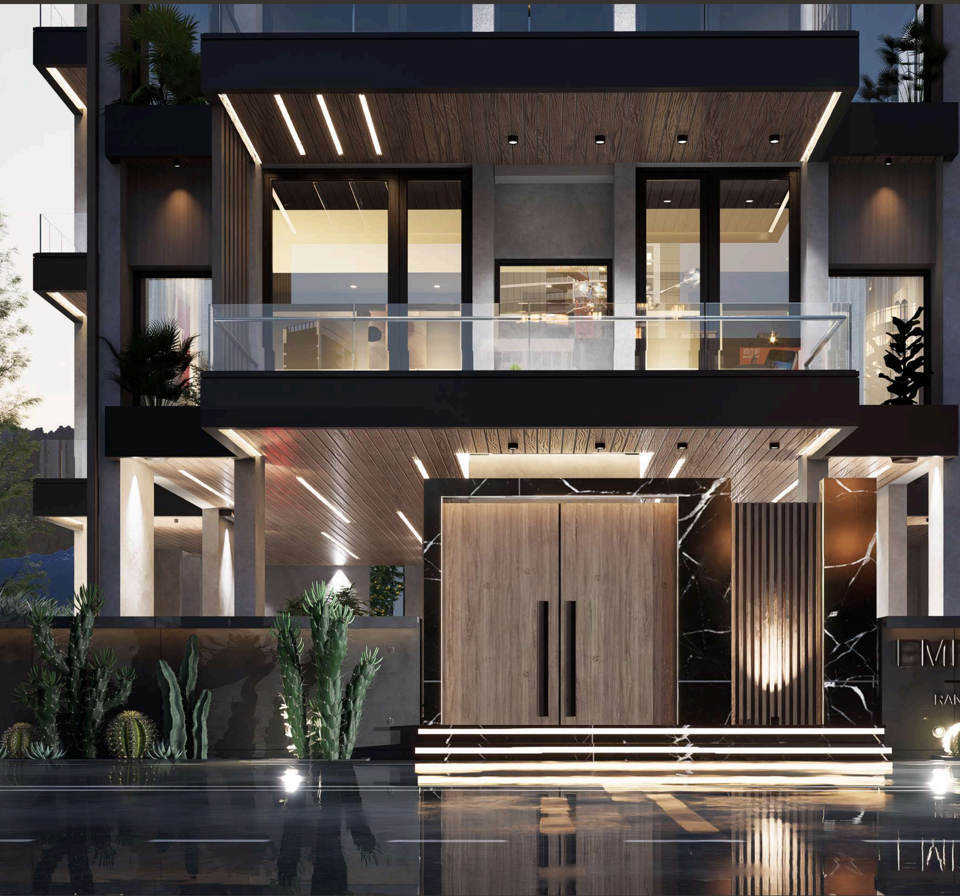
Main Facade Entrance
