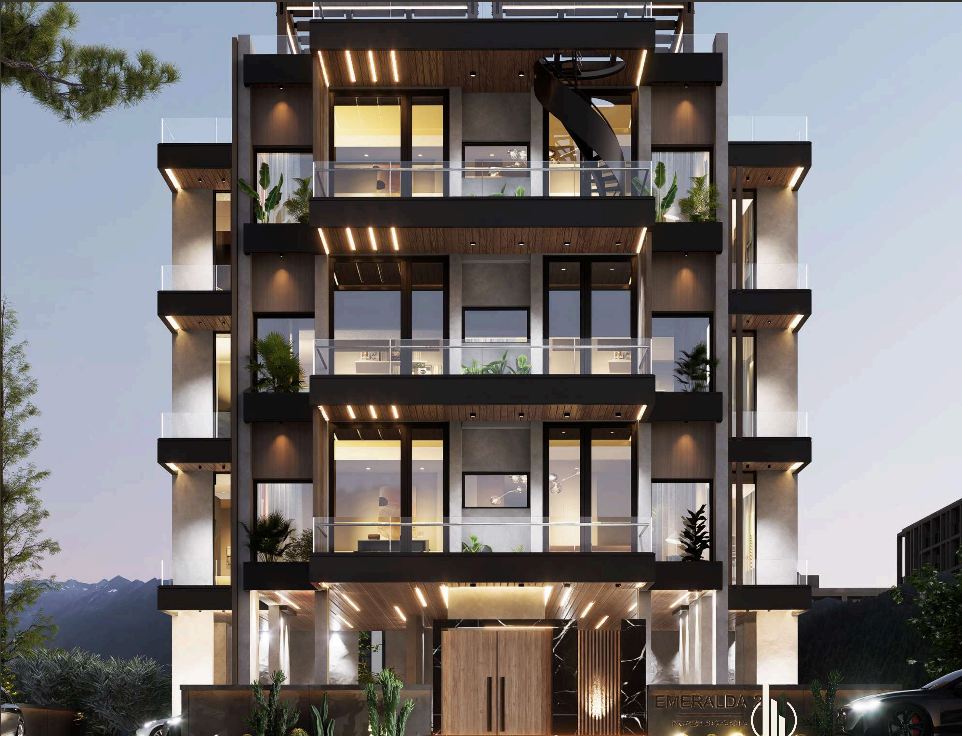
Facade Wide View
